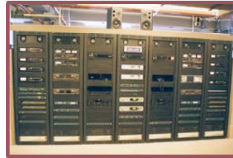
Completed equipment racks.
